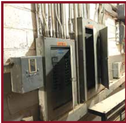
This rule is followed by the maintenance men at a Texas high school: Never stand in front of a breaker panel when turning breakers on or off. Be sure to stand next to the panels, out of the way.
